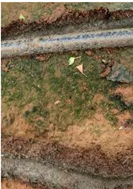
Fine clay particles around the dripper line and fine roots forming a mass which will eventually restrict water flow.
